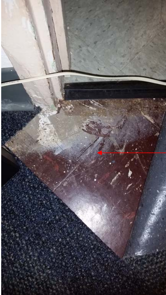
Photograph 1: 9"x9" Brown Vinyl Floor Tile (VFT) under carpet and 12"x12" Gray Speckled VFT.
